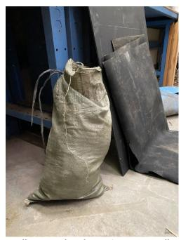
Sandbags used under Weirs  $\sim 30-40$  lbs.; fills and empties sandbags on the riverbank to minimize the distance they are carried.
