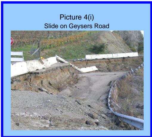
Repairing washouts- As with slides, the first step is debris removal. Then the toe of the embankment is excavated, and the embankment is reconstructed. Proper drainage must be installed, or existing drainage repaired, to prevent future washouts. Damaged roadway features, including pavement and base/sub-base, guardrail, and signs or markers, are repaired or replaced. The area may also be re-vegetated or buttressed with rock or walls to protect steep natural slopes.
