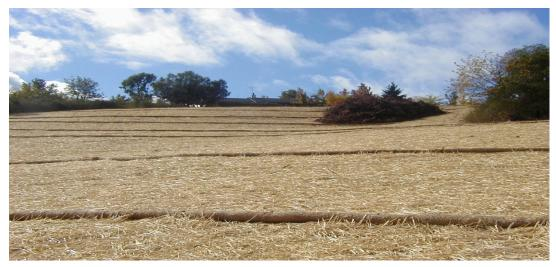
Straw wattles or fiber rolls are designed to slow down runoff, filter and trap sediment before the runoff gets into watercourses. Straw wattles are porous and allow water to filter through fibers and trap sediment. They also slow down runoff thereby reducing sheet and rill erosion.
