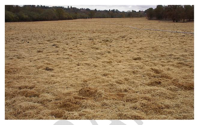
The most effective erosion control practice (both in terms of protection and cost) is the use of cover crop and straw mulch. Straw provides a cushion between the disturbed soil and the velocity of the raindrop. It's the best insurance for **protection** from the early rains if you cannot plant your cover crop in mid-September and irrigate it.
